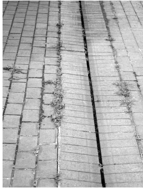
Plants in mortar joints on Cromwell Highwalk
