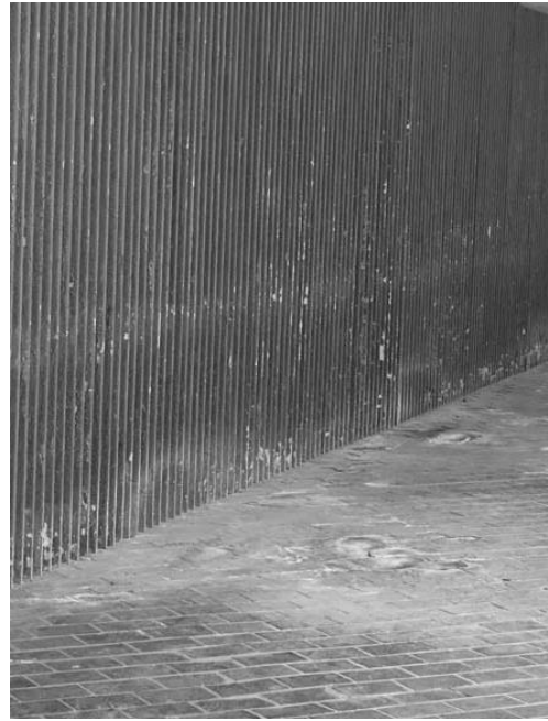
Railings unpainted for at least 20 years and 20 mm thick calcination on Defoe Place
